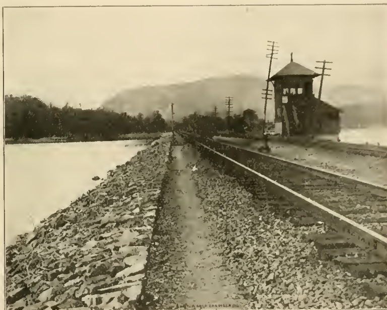
TYPICAL RAILWAY BLOCK SIGNAL TOWER.
